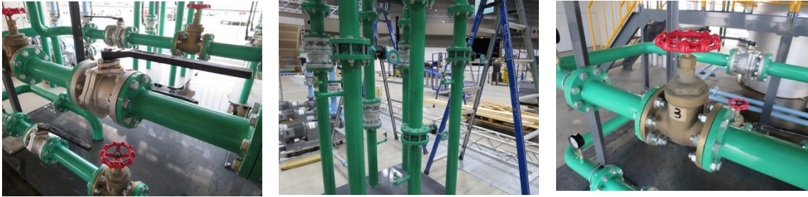
From left: Ball Valve, Rubber Seated Valve, Gate Valve
